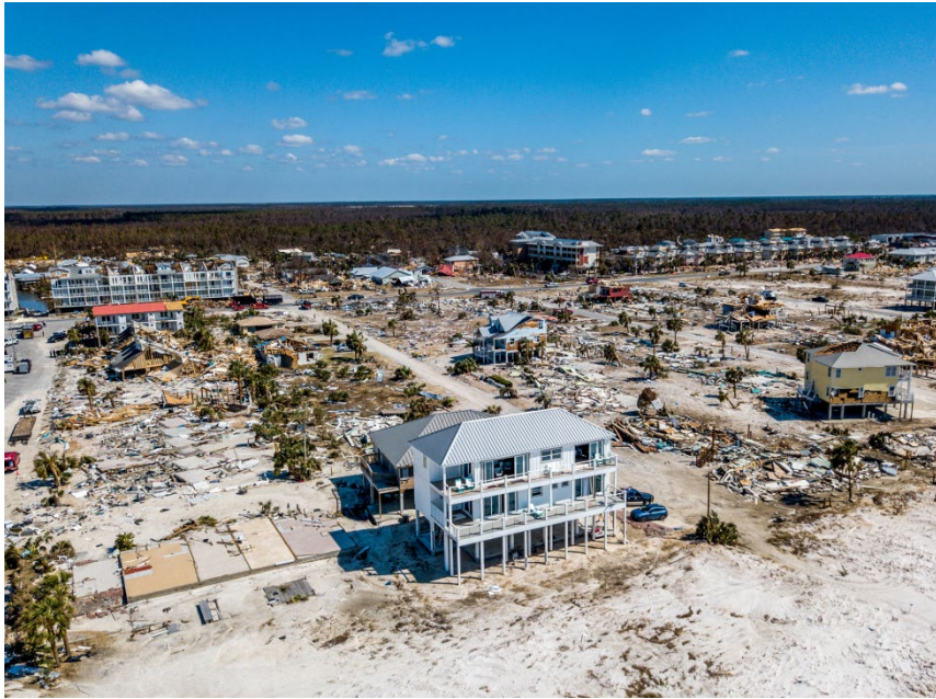
Hurricane Michael (2018) Florida, Mexico Beach, USA
